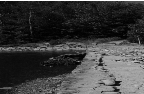
Ravine House Pool Dam- 2011 Overflow Damage photo credit: Gail Scott
